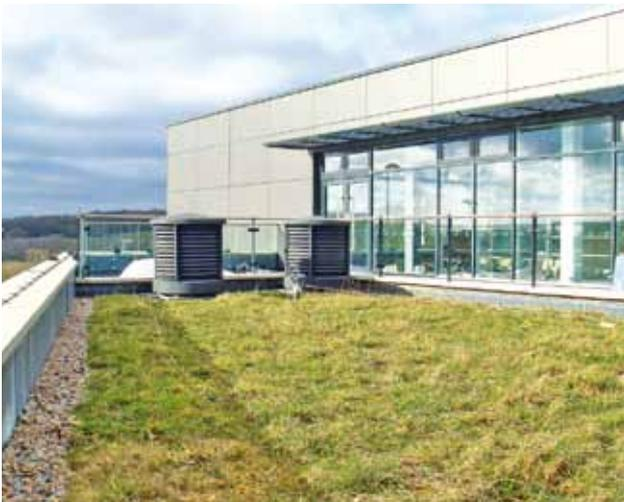
The Sussex Exchange is covered with green and brown roofs integrating ventilation and infiltration. Within the brown roof parts the environmentally diverse brown field sites were replicated and thus, vegetation associated with such sites can colonise a range of low-fertility substrates.
